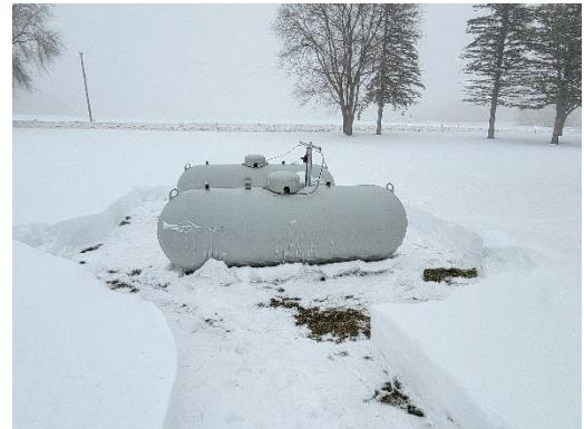
#1 Properly cleared access to tanks
